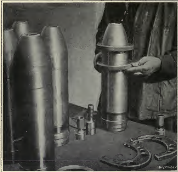
Fig. 89. Gaging External Diameter and Thread In Nose
