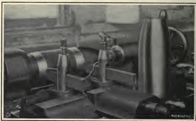
Fig. 101. Turning External Diameter to Size and Shape
