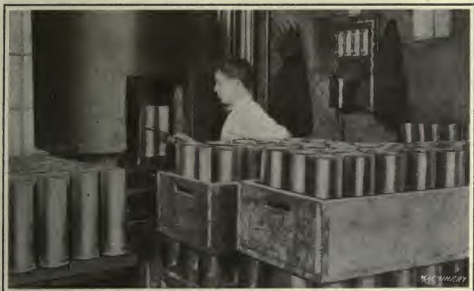
Fig. 152. Annealing Mouth in a Special Furnace previous to tapering
