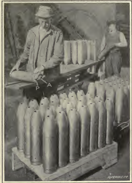
Fig. 93. Gaging Concentricity of Shell
