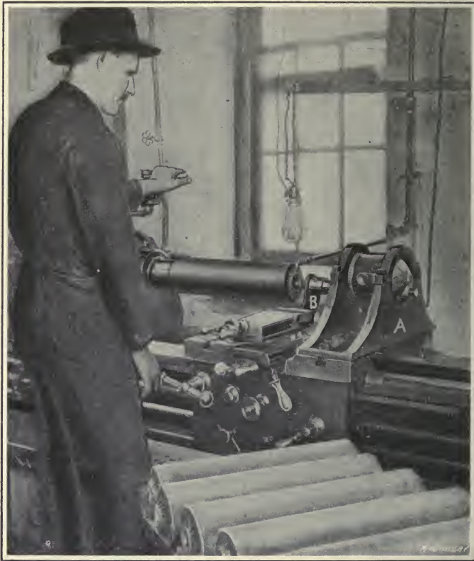
Fig. 72. Centering Closed End of Forging
