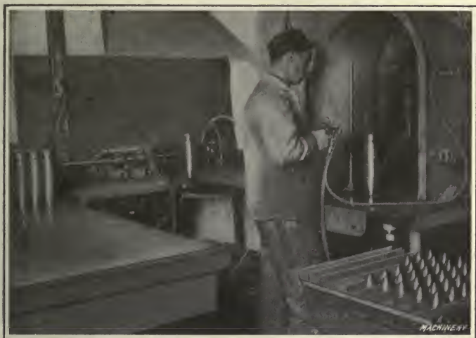
Fig. 63. Spraying Interior and Exterior of Shell with Copal Varnish
