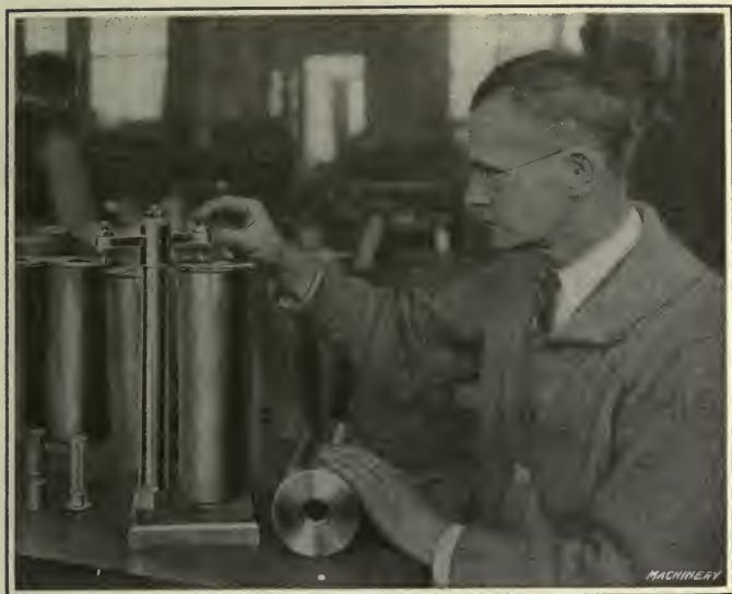
Fig. 156. Gaging Thickness of Head of Cartridge Case
