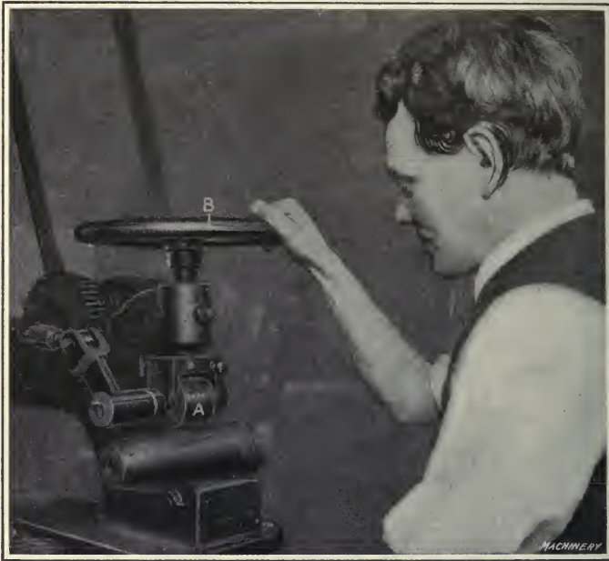
Fig. 38. Stamping in a Holden-Morgan Rotary Stamping Machine
