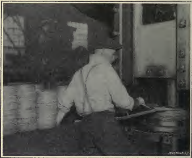
Fig. 140. First Operation—Cupping In a Toledo Press
