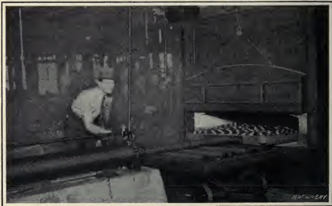
Fig. 170. Annealing Cartridge Cases In a Quigley Oil Furnace for Thirty-five Minutes
