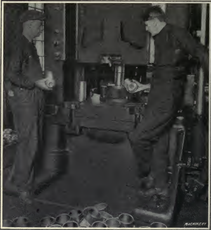
Fig. 148. Second Indenting Operation on a Toledo Press
