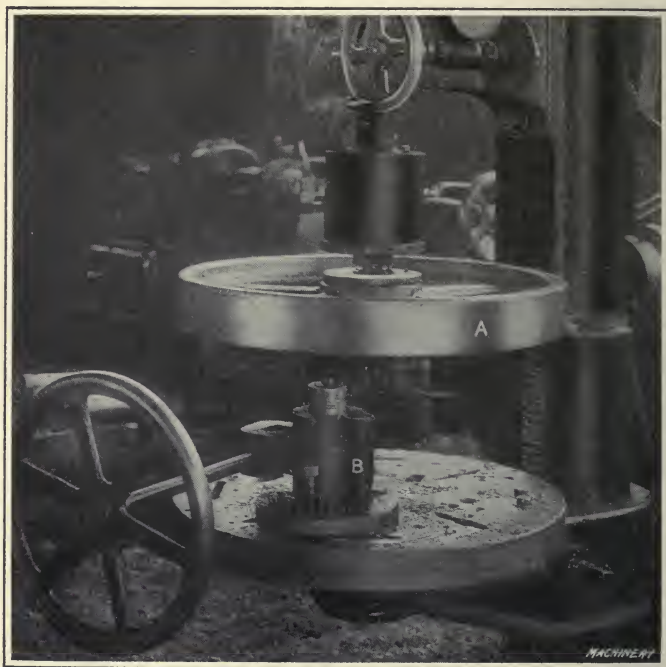
Fig. 47. Fixture used for driving in Gas Plugs
